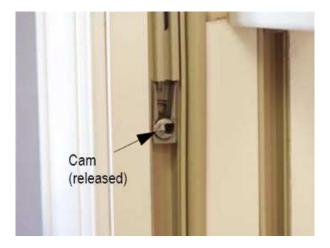
Rotate the balance clutch cam to the open locked position (cam opening up). Release the screwdriver carefully from the clutch assembly (it must lock in place or damage will occur).
